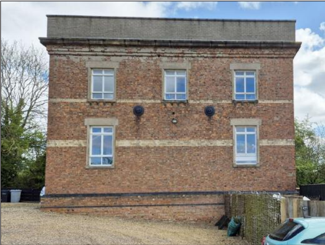
The Water Tower built about 1880 to supply water to the steam engines on the nearby railway.
